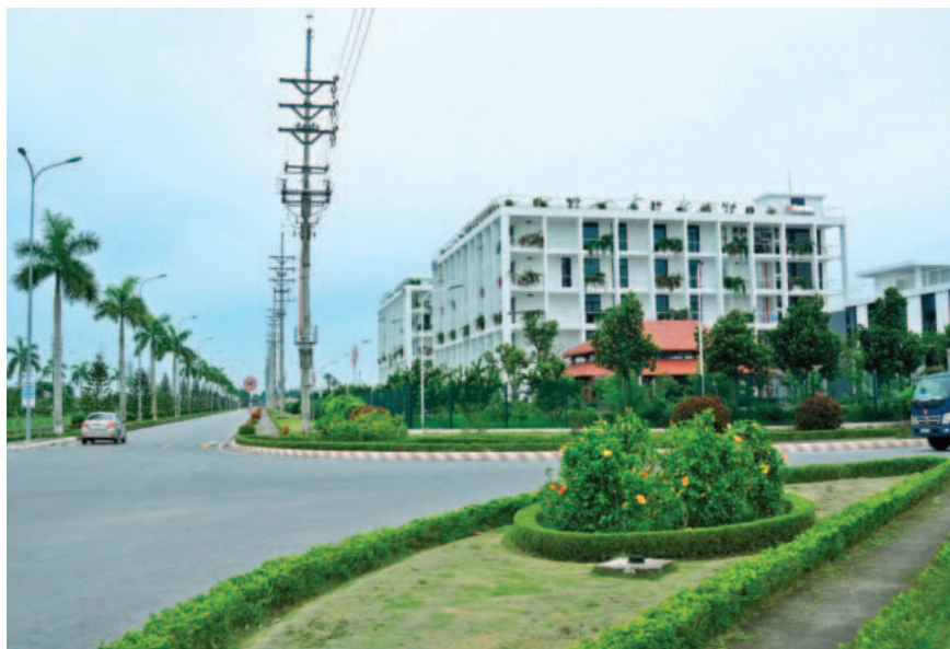
Projects in Thang Long Vinh Phuc Industrial Park are designed with a focus on environmental sustainability and utilize cutting-edge technology
