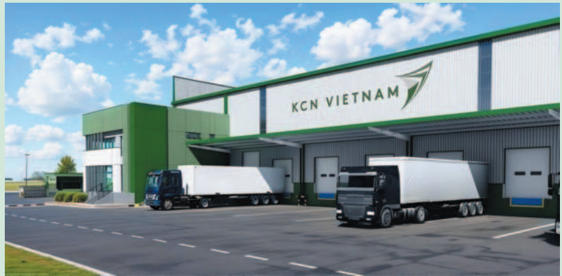
Projects that adhere to green standards, such as KCN DEEP C - Hai Phong (Phase 02) by KCN Vietnam Group, aim to ensure a balance between environmental and economic efficiency
