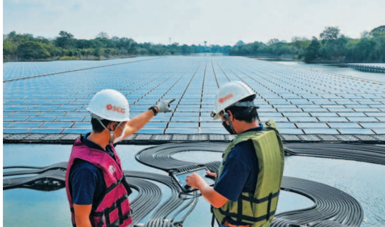
SCG’s smart grid intelligent network for clean energy management
